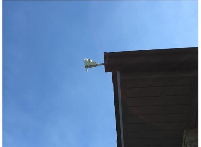
PROPER INSTALLATION OF A RAIN SENSOR
