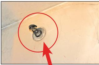
These types of heads are usually seen on the side of a wall, not overhead. Although there are also types of heads that can be placed overhead as well. These are usually installed in areas where temperatures are subject to freezing.
